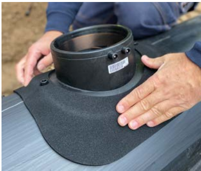
The self-adhesive rubber mat seals the saddle on an ASA VL d160 pipe.
