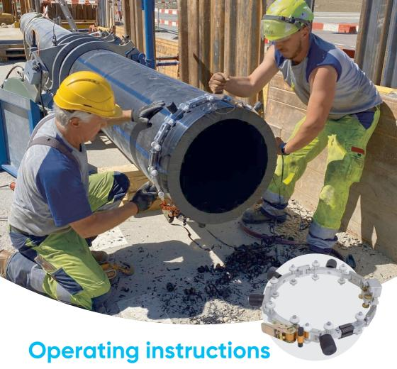
Chain Peeler for the use of PE – and PP – pipes d 250 – 1000 mm / 10 – 36 "IPS / 10 – 36 "DIPS
