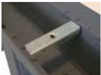
Grate locking device applicable (pag. 198)
